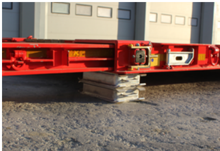
Placing the supports under the pool
